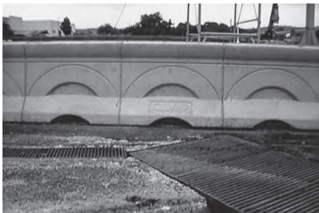
Figure 5. New Jersey barrier used in Rome.
