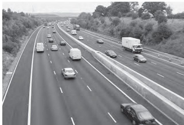
Figure 7. Concrete barriers used in the United Kingdom.
