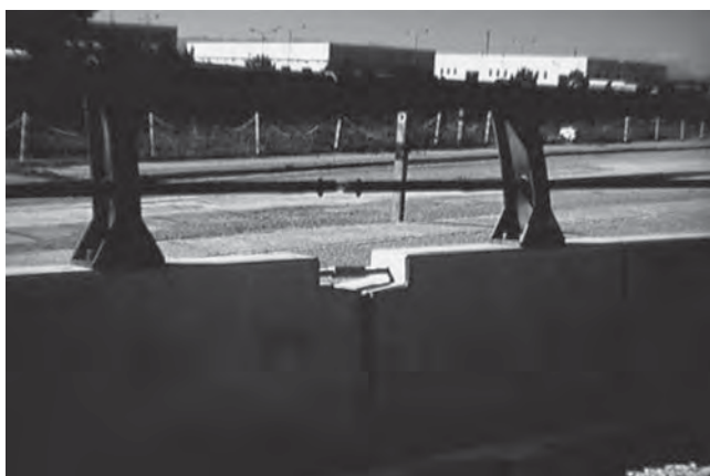
Figure 6. New Jersey border bridge used in Italy.
