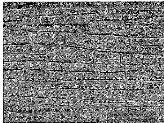
Dry stacked rock design was recently crash tested and received approval for use in California.
